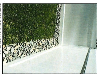
RIVER STONE PAVING UNDER FENCE
