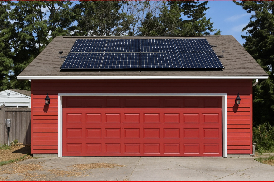
EXAMPLE OF A GARAGE WITH SOLAR PANELS
