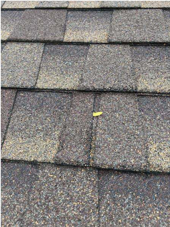
Roof Information / Photo: Roof Condition
