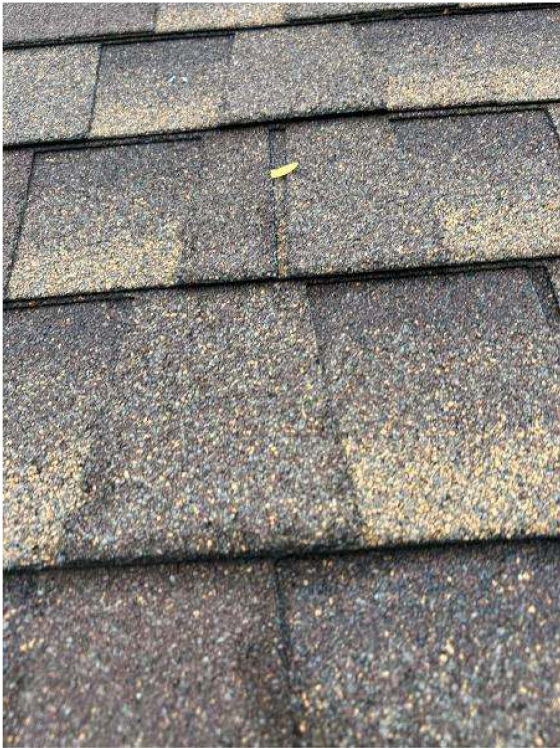
Roof Information / Photo: Roof Condition
