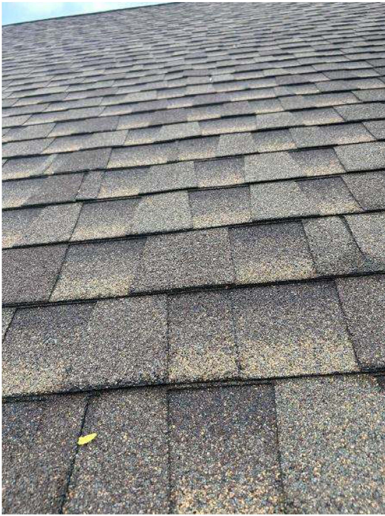
Roof Information / Photo: Roof Condition
