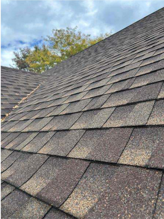
Roof Information / Photo: Roof Condition
