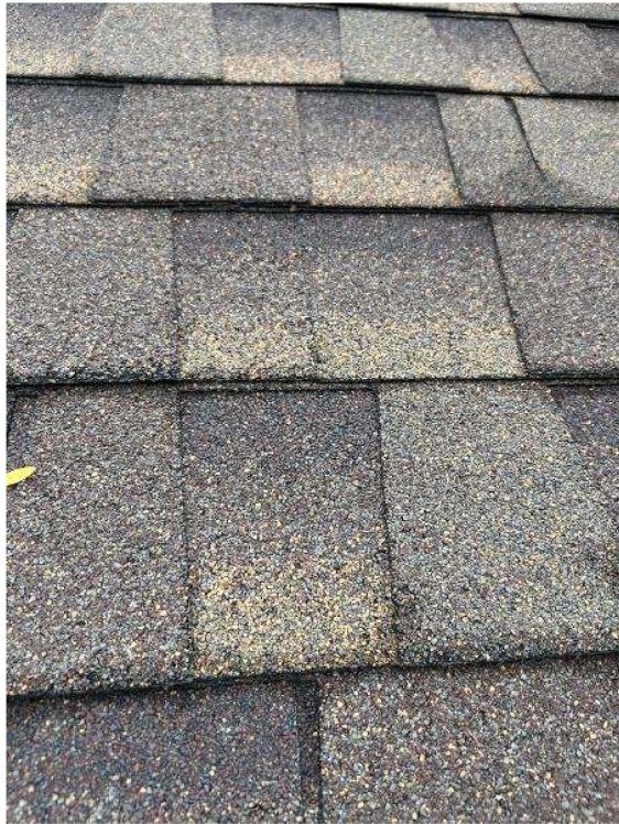
Roof Information / Photo: Roof Condition
