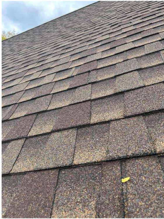
Roof Information / Photo: Roof Condition
