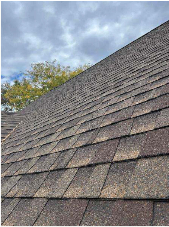
Roof Information / Photo: Roof Condition
