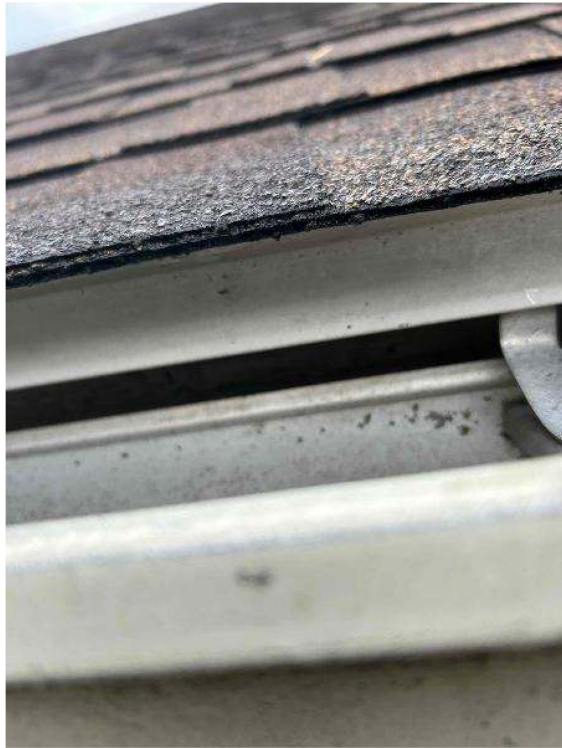
Roof Information / Photo: Roof Condition
