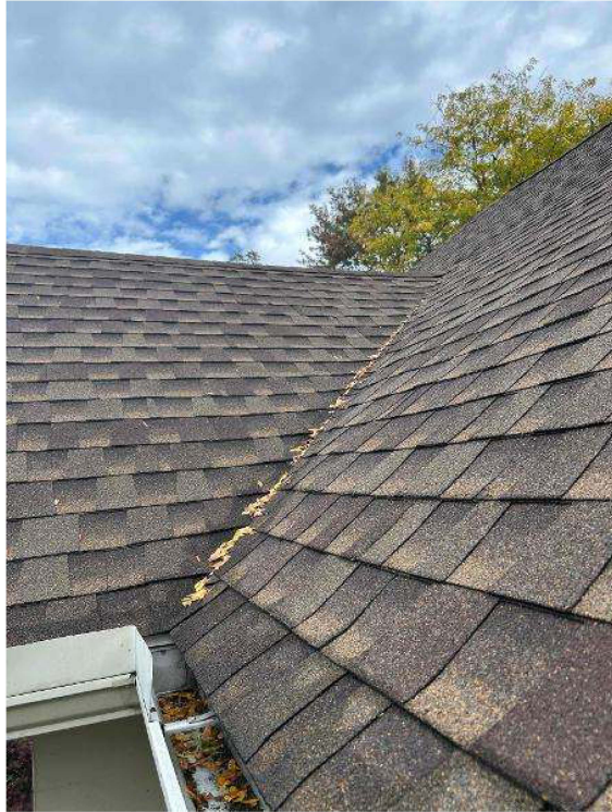
Roof Information / Photo: Roof Condition
