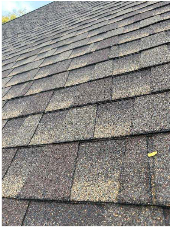
Roof Information / Photo: Roof Condition
