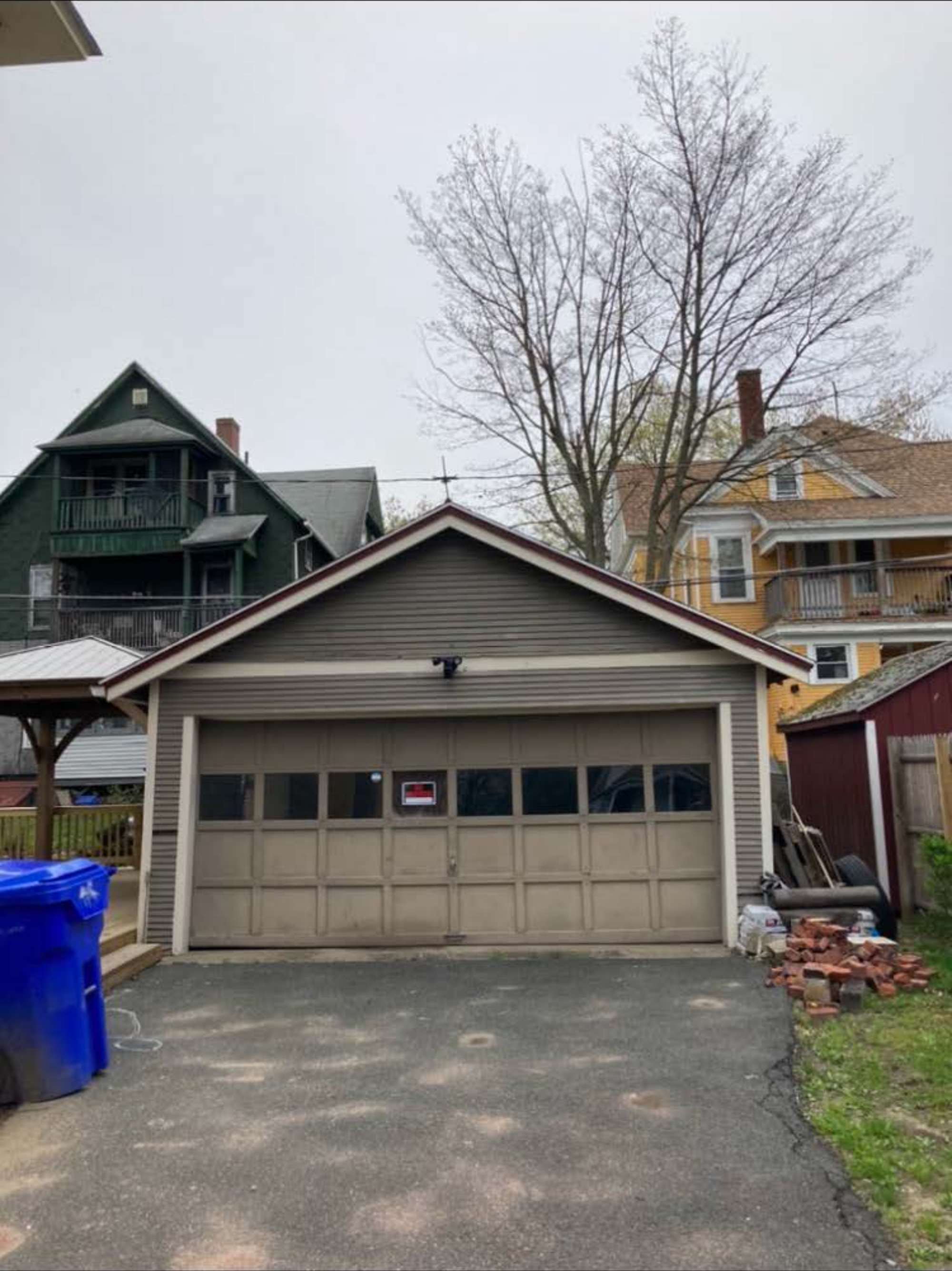
Detached garage with accessible opening on left side.
