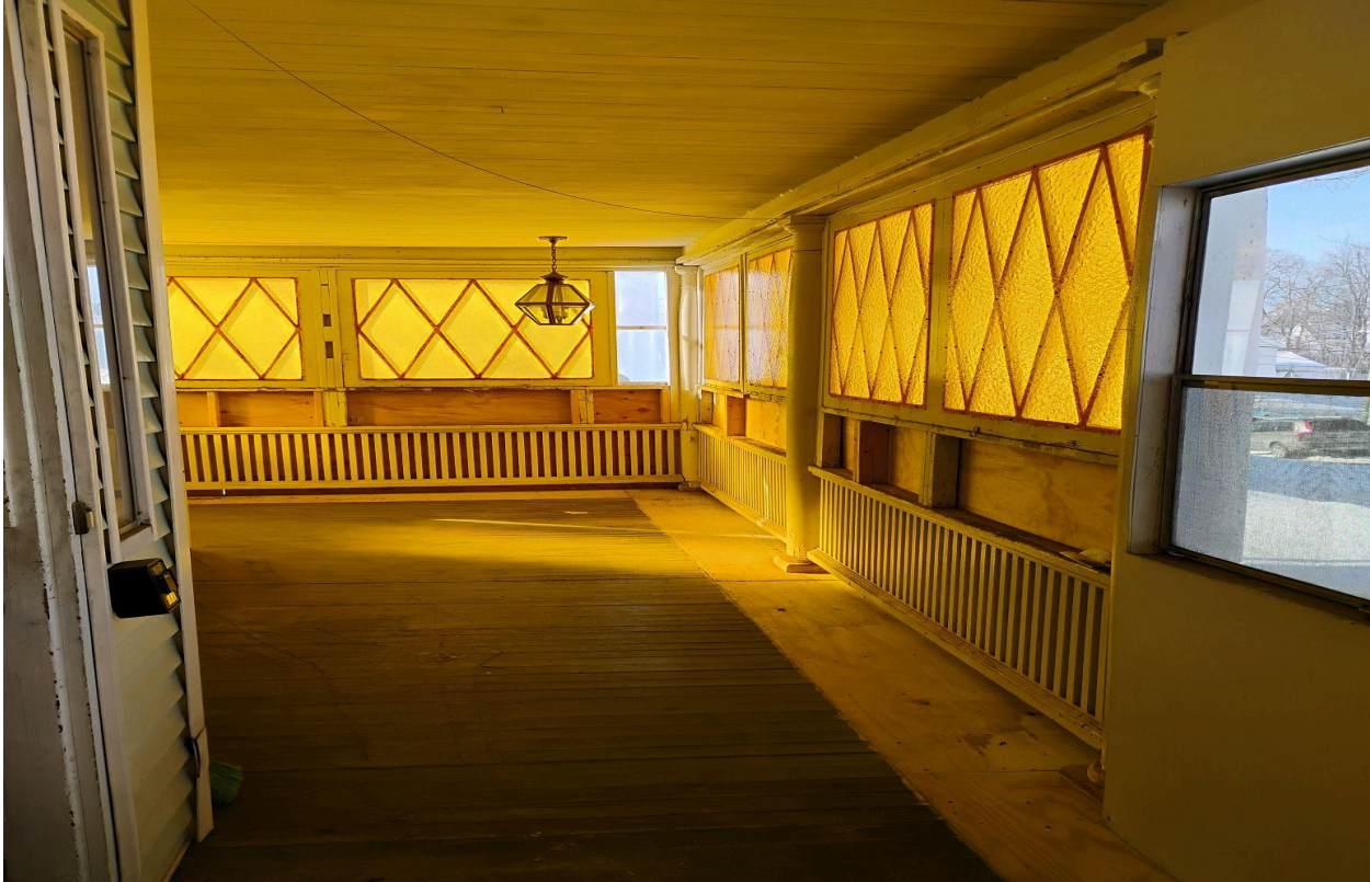
Restoration of historic open porch: reverting to original 1905 design
