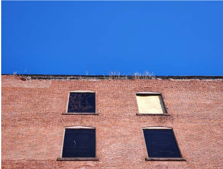
Photograph #38 – Exterior Masonry at Roof Edge
