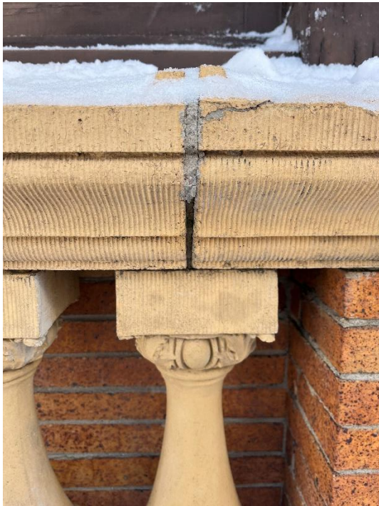
Mortar gaps, cracked balustrades, and rooftop location of additional balustrades
