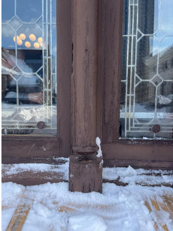
Examples of window trims in need of repair and repainting.
