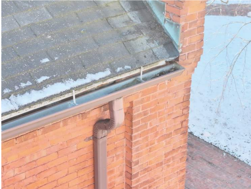
14. View of Parish House non-historic gutter eave and downspout.
