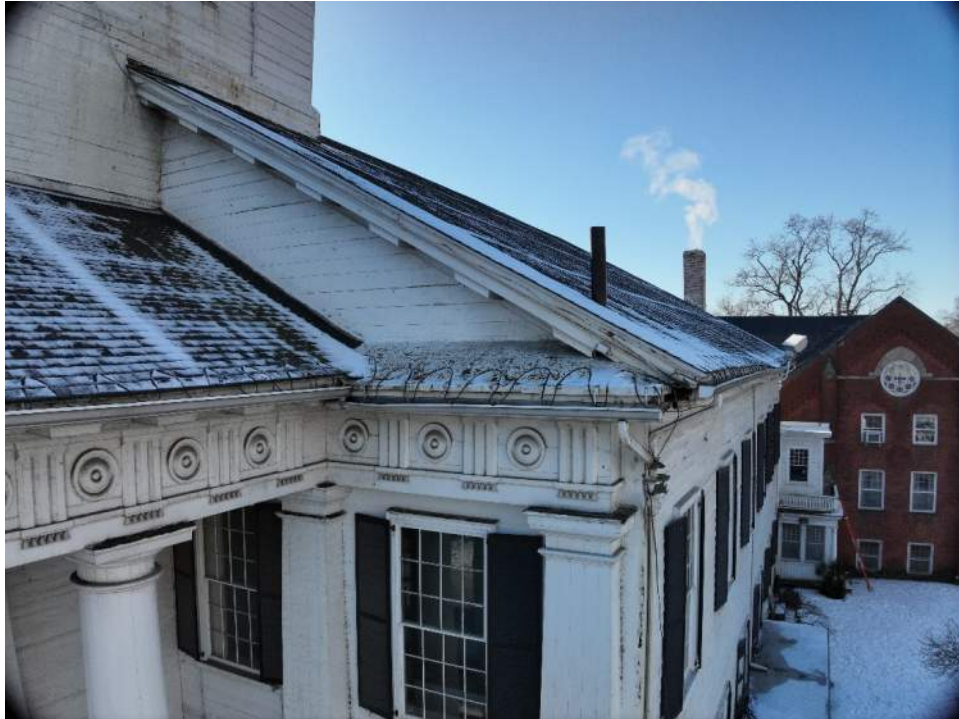
10. Partial elevation of the northeast corner of the Church roof eave, rake, and soffit.
