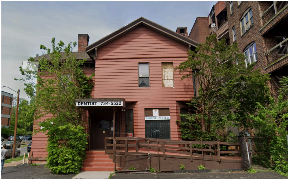
Window on front of property repaired without a building permit.
