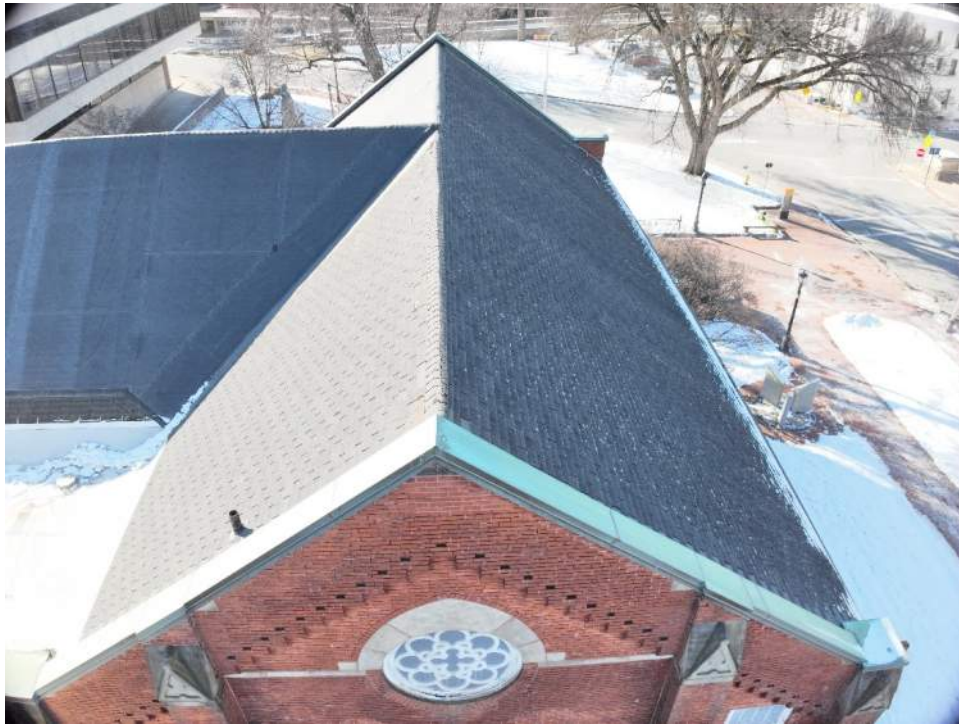
15. Parish House north wing existing strip asphalt shingles.
