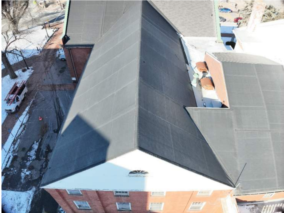
16. Parish House south wing existing EPDM (single-ply rubber) roof covering.
