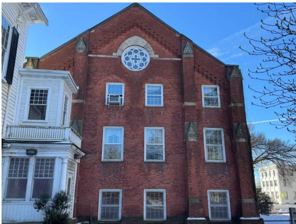
6. Partial east elevation of the Parish House.
