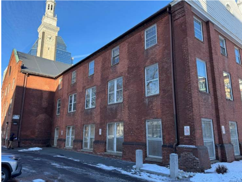
8. Partial west and south elevations of the Parish House.
