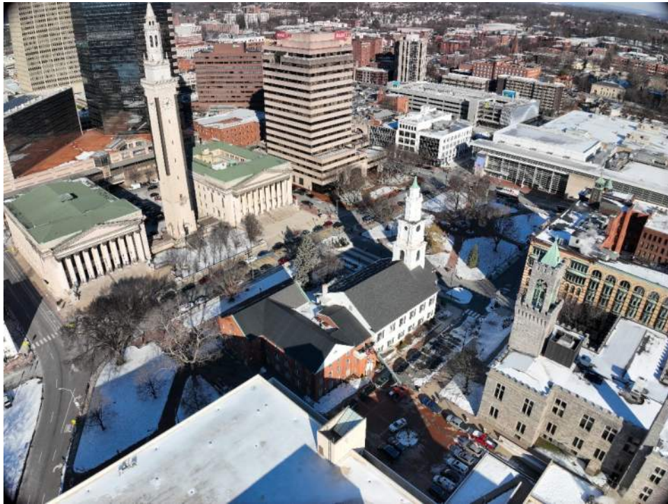
3. Photo 3 – View of the Old First Church looking northeast
