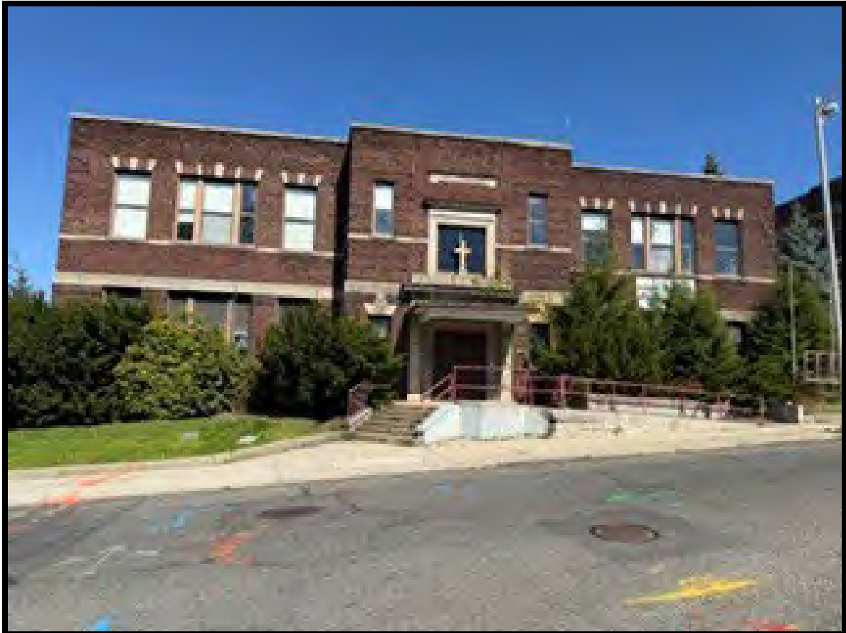
Site A 334 Franklin Street, Springfield, MA
