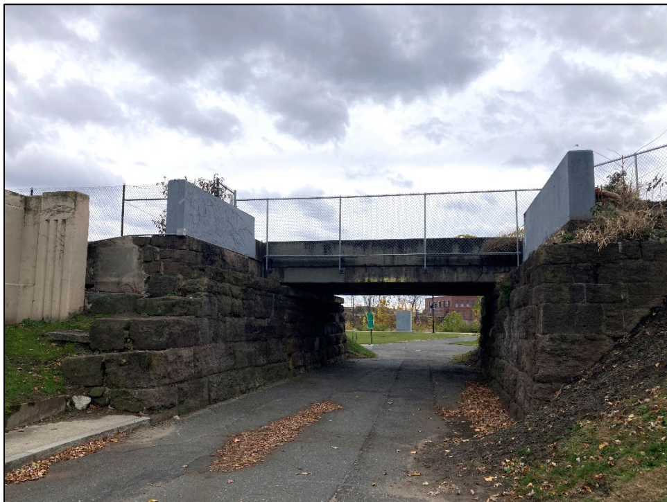
Photo 2. Elm Street Bridge, view facing southwest (11/13/25).
