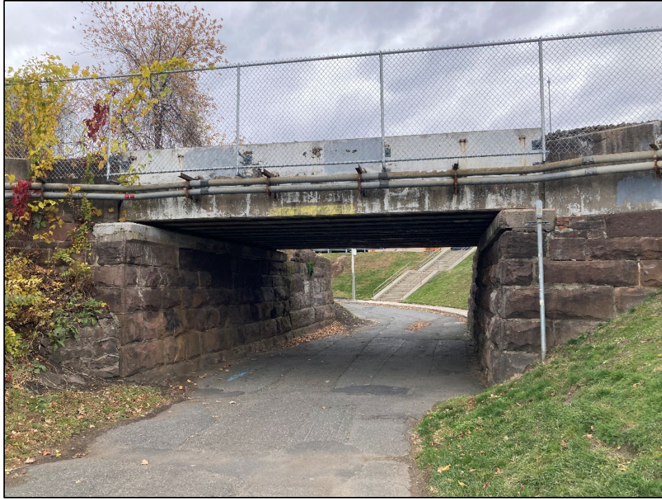
Photo 3. Elm Street Bridge, view facing northeast (11/13/25).
