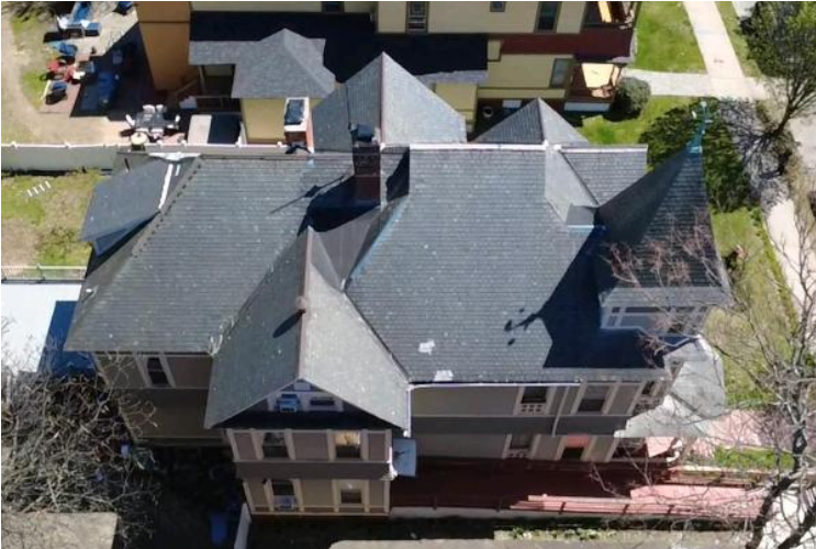
Exterior Evaluation / Exterior Home Structure Walls
