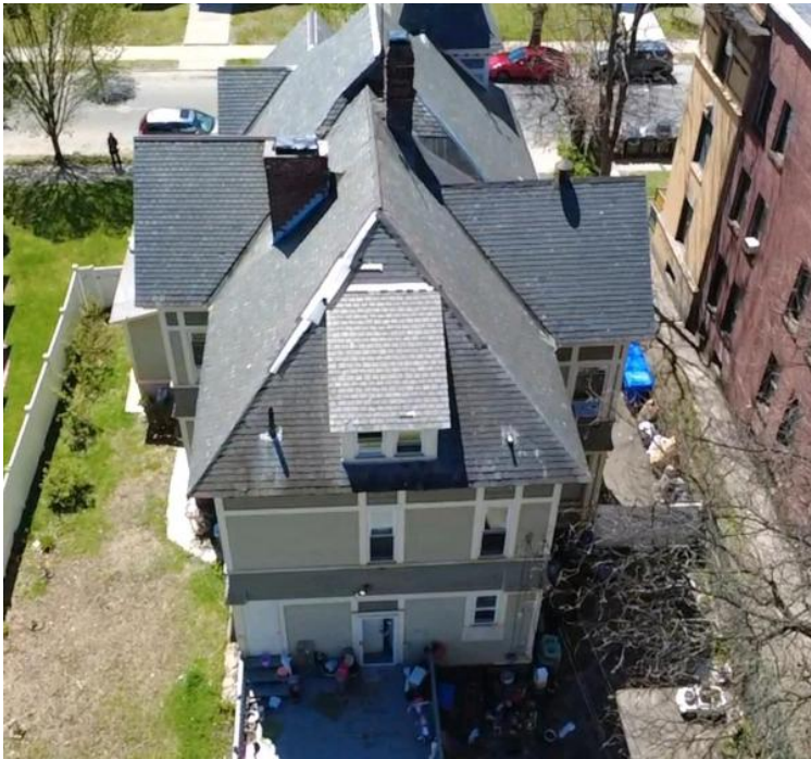
Exterior Evaluation / Exterior Home Structure Walls
