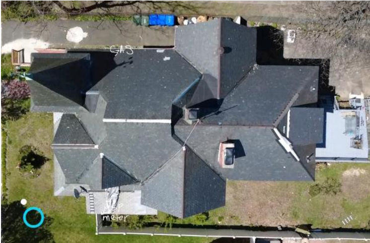
Exterior Evaluation / Exterior Home Structure Walls
