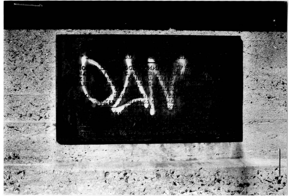
ON N END PARAPET, SPRINGFIELD SIDE (2-28-1985)
