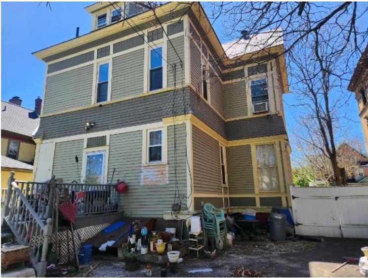
Exterior Evaluation / Exterior Home Structure Walls
