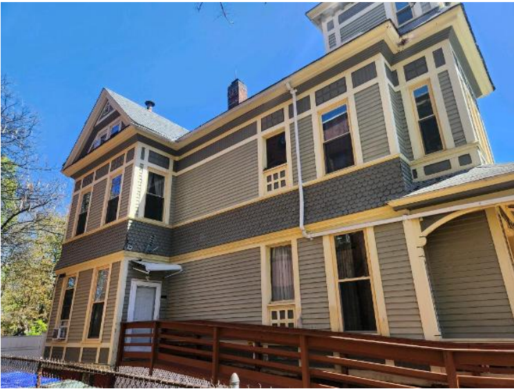
Exterior Evaluation / Exterior Home Structure Walls
