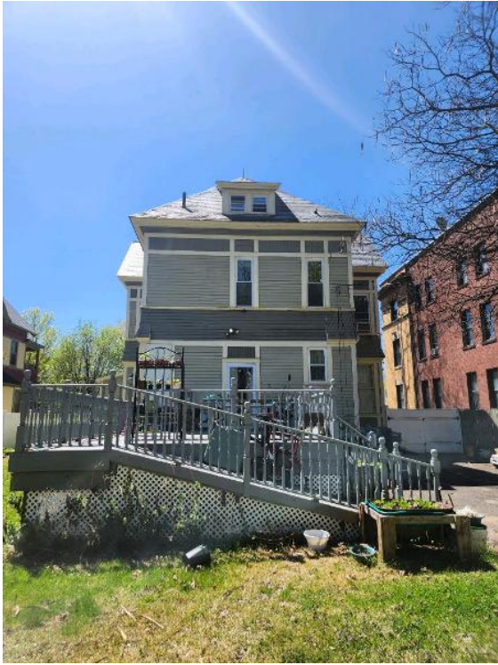
Exterior Evaluation / Exterior Home Structure Walls
