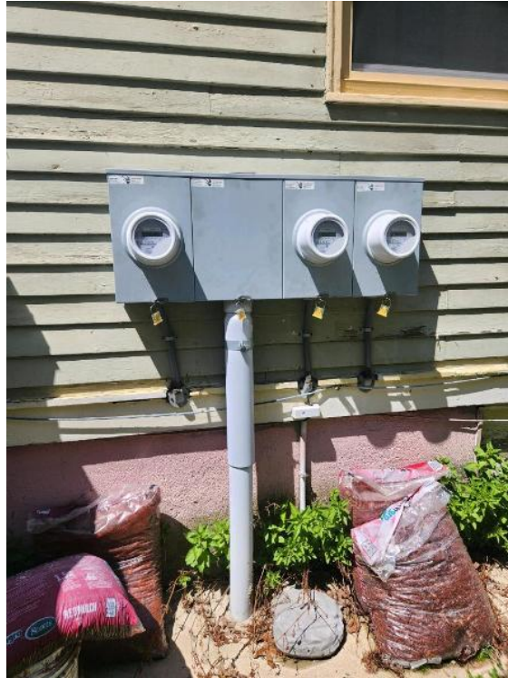
Electrical Evaluation / Meter/Main Combo
