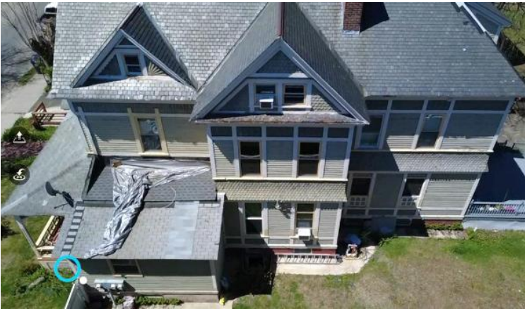
Exterior Evaluation / Exterior Home Structure Walls
