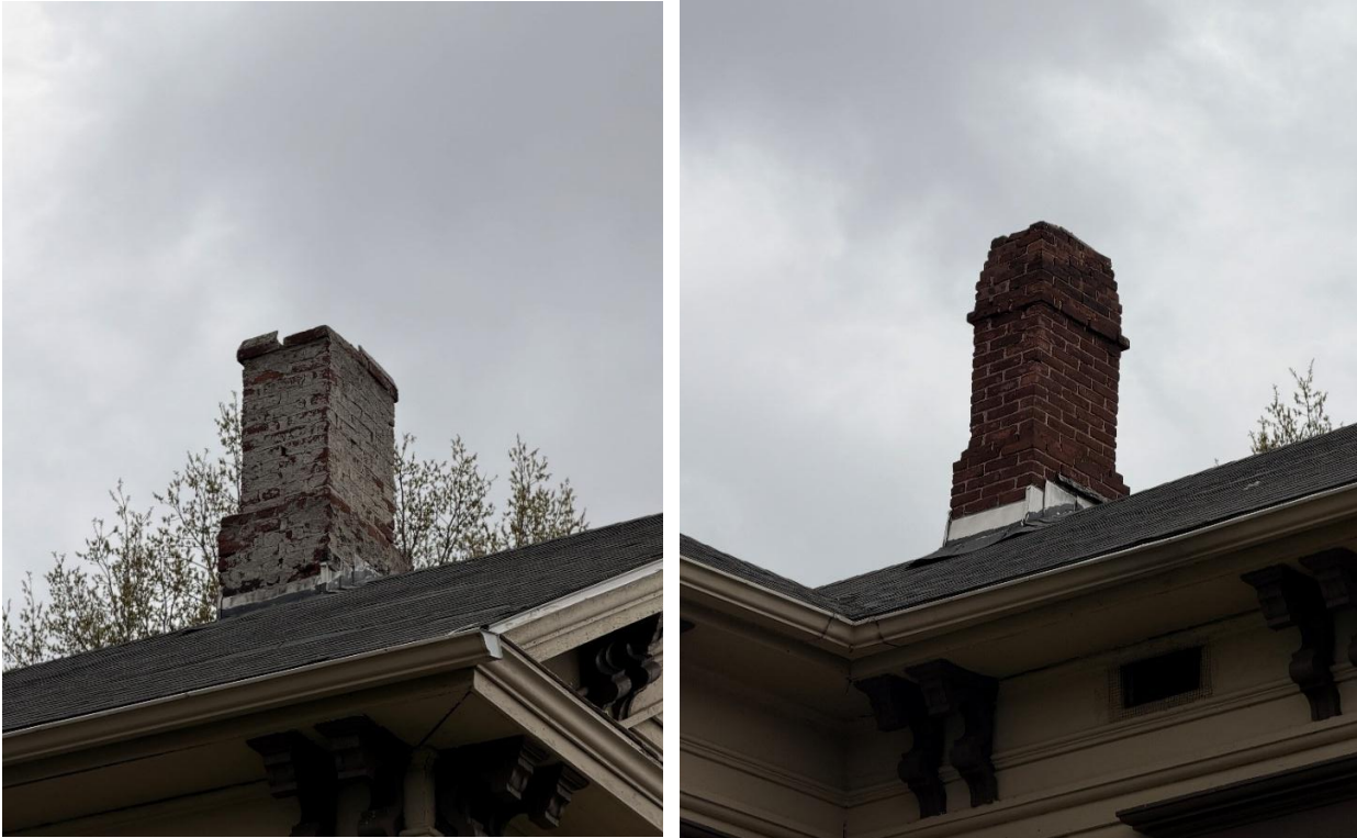
Fig. 7: Existing Chimney Condition
