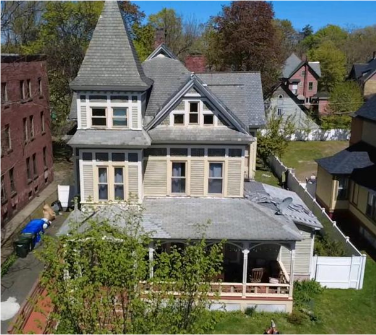
Exterior Evaluation / Exterior Home Structure Walls
