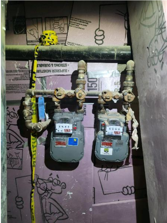
Exterior Evaluation / Gas Meter
