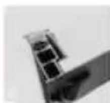
Anti-theft alarm frame and thermal break . Expanded polystyrene is going to insulate the gap
