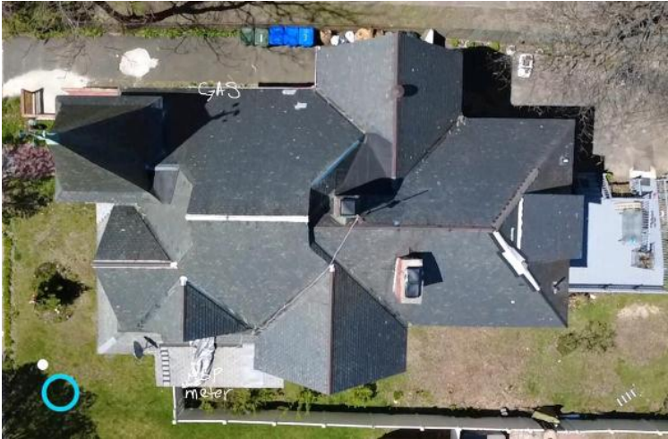
Electrical Evaluation / Distance From Meter to MSP
