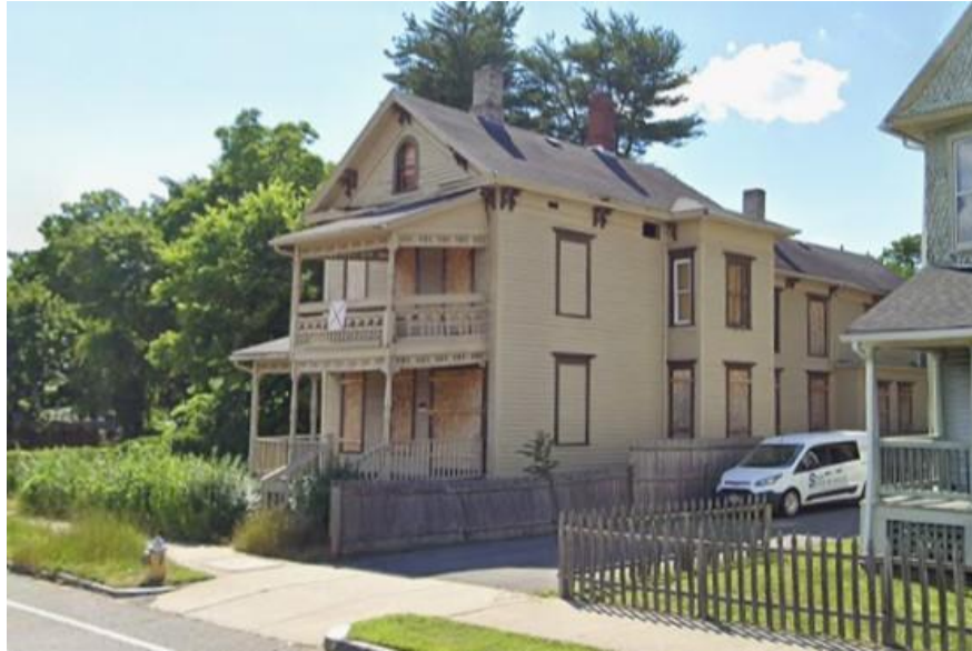
Fig.4: Southeast corner from Bay St.
