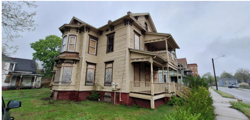
Fig.5: Southwest corner from Bay St.
