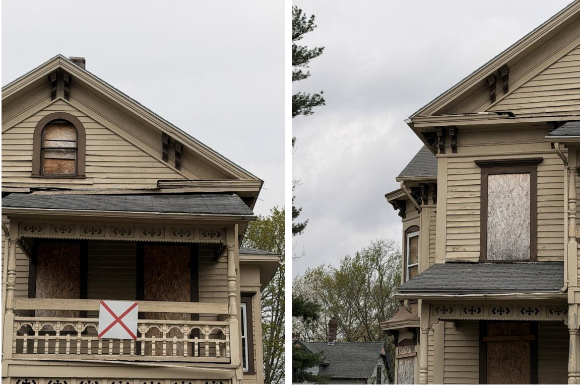
Fig.6: Existing Roof Condition
