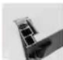
Anti-theft alarm frame and alarm cover with thermal break . Expanded polystyrene is going to insulate the gap
