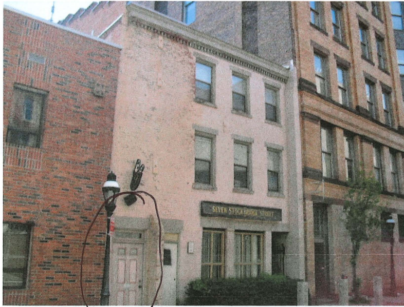
Note wood panel door in circa 2012 photo
