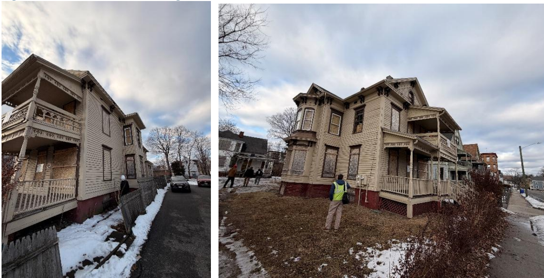
Fig. 2: Left – Southeast Elevation, Right – Southwest Elevation
