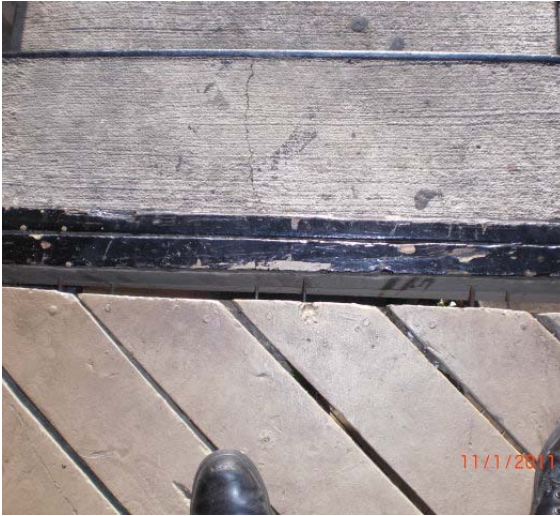
Stairway being held up only by nails and pulling away from walkway.
