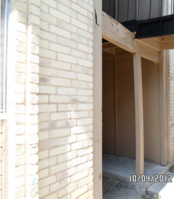
Sagging horizontal member beam and bowing support post not strong enough to carry imposed load.
