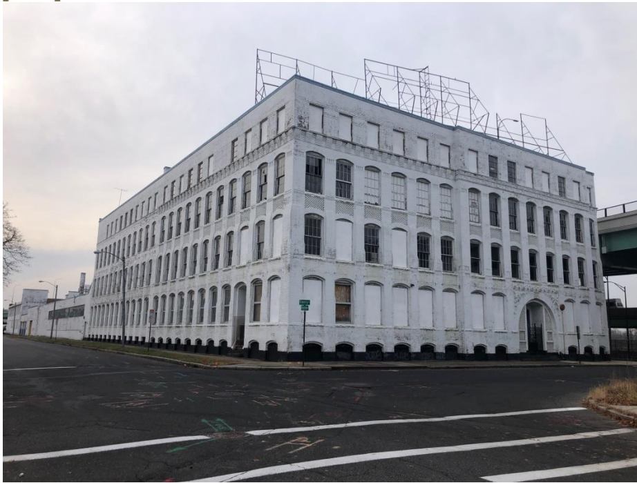
Photo 1: Corner of Emery Street and Boylston Street
