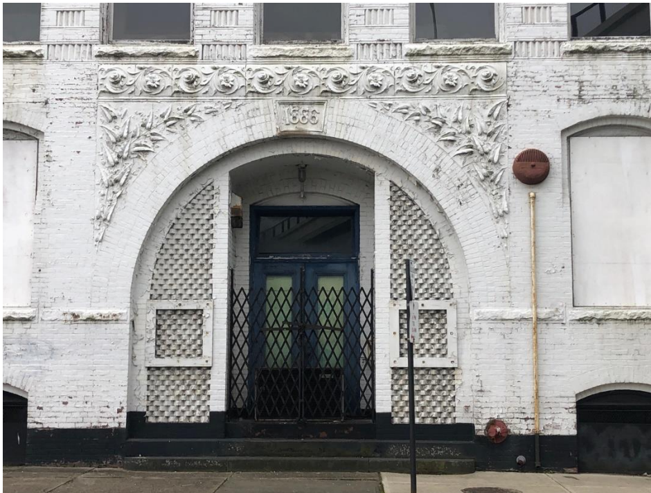
Photo 2: Emery Street entrance
