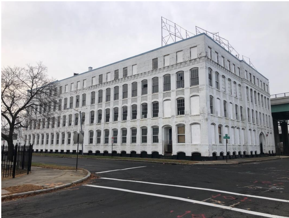
Photo 4: Corner of Emery Street and Boylston Street
