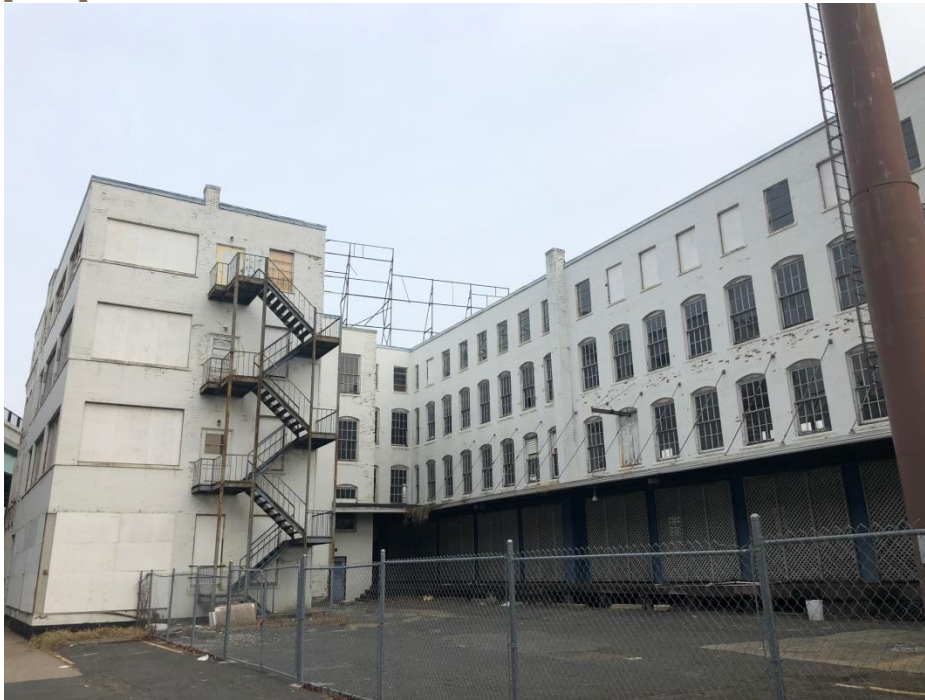
Photo 3: Elevation along East Columbus Ave near the corner of Emery Street
