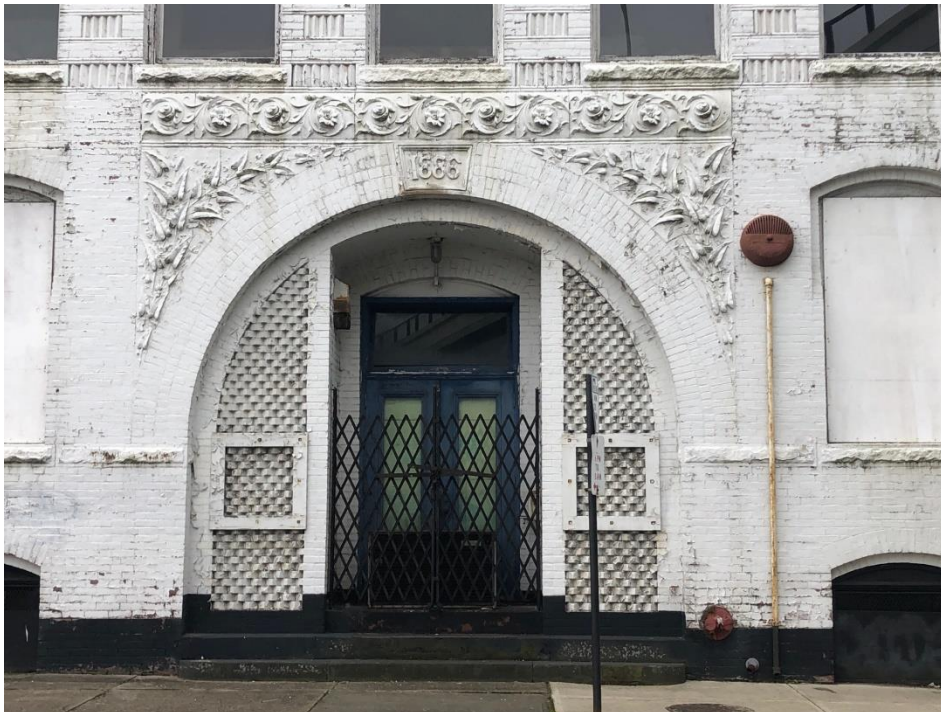
Photo 2: Emery Street entrance
