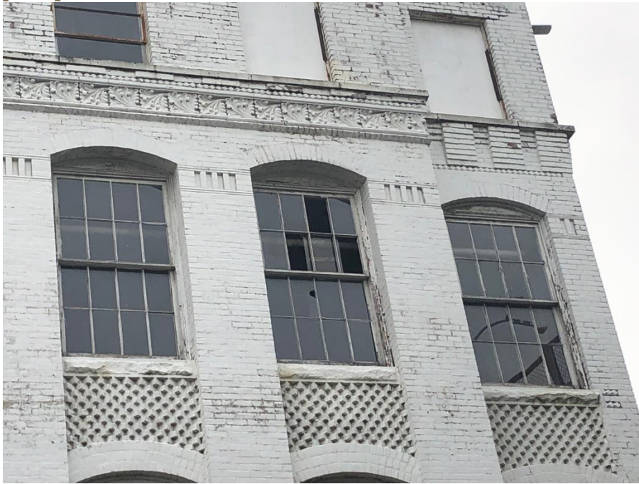
Photo 5: Emery Street Façade showing architectural details
