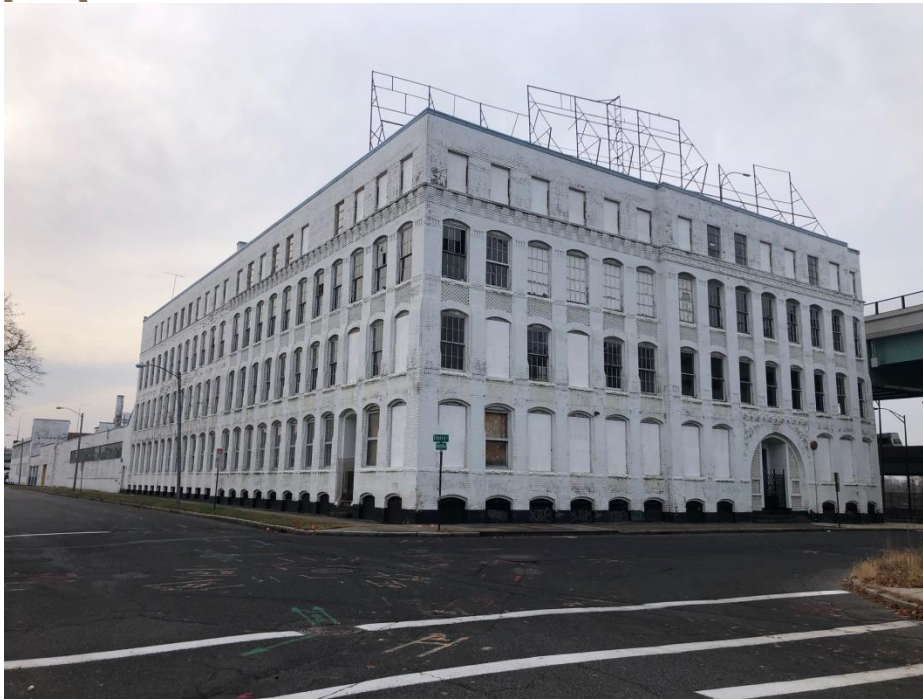
Photo 1: Corner of Emery Street and Boylston Street
