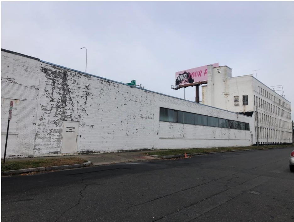
Photo 6: Elevation along Boylston Street showing later addition
