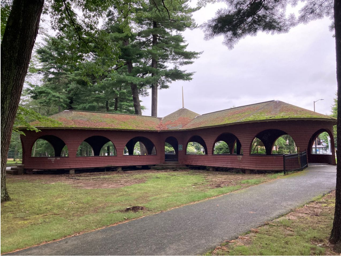
Photo 3: Forest Park waiting pavilion, exterior view looking northwest.
