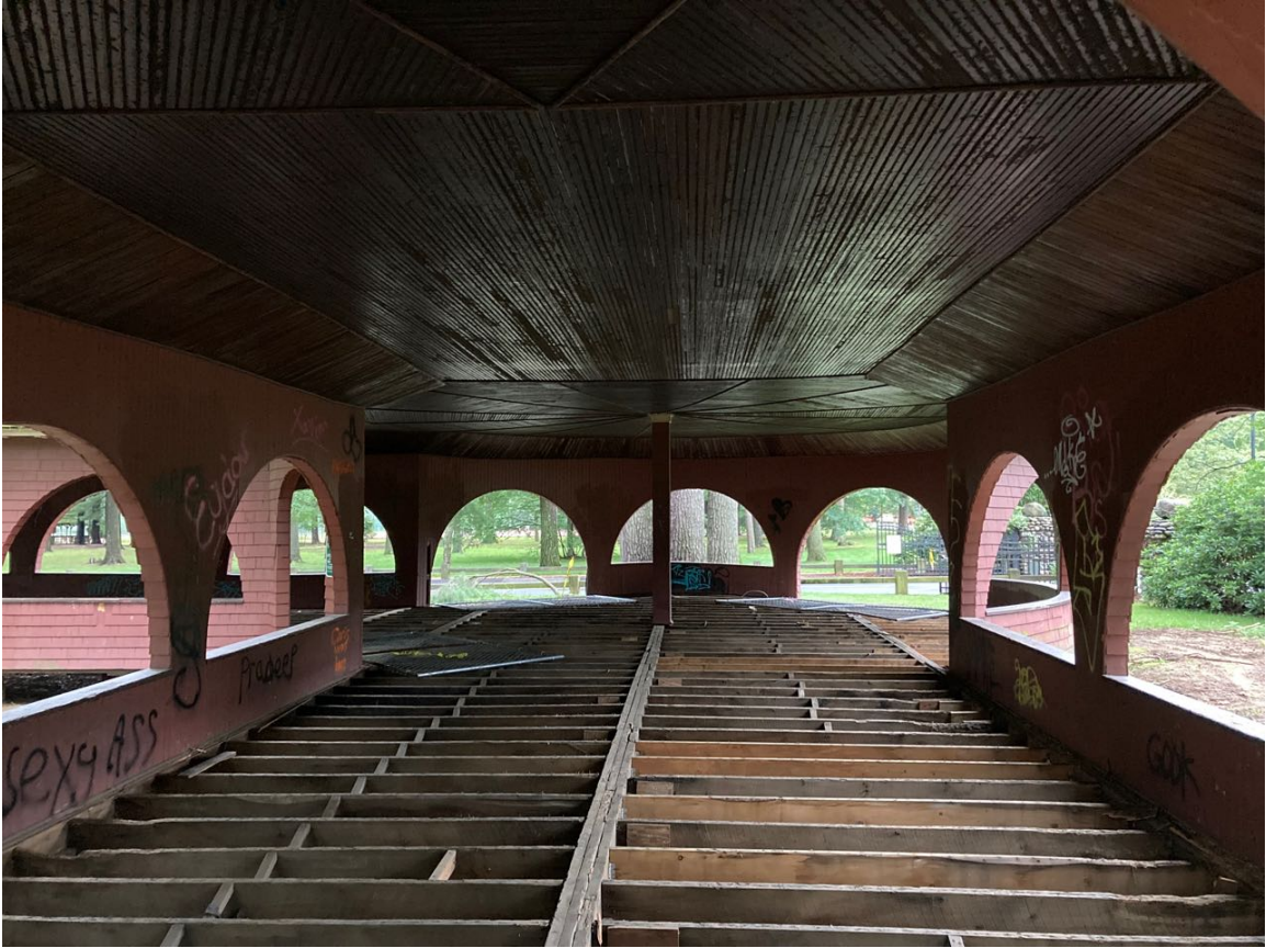
Photo 7: Forest Park waiting pavilion, interior view looking west.
