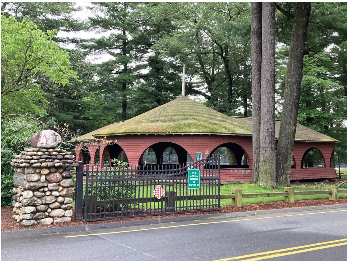
Photo 1: Forest Park waiting pavilion, exterior view at park entrance, looking southeast. (1660)
