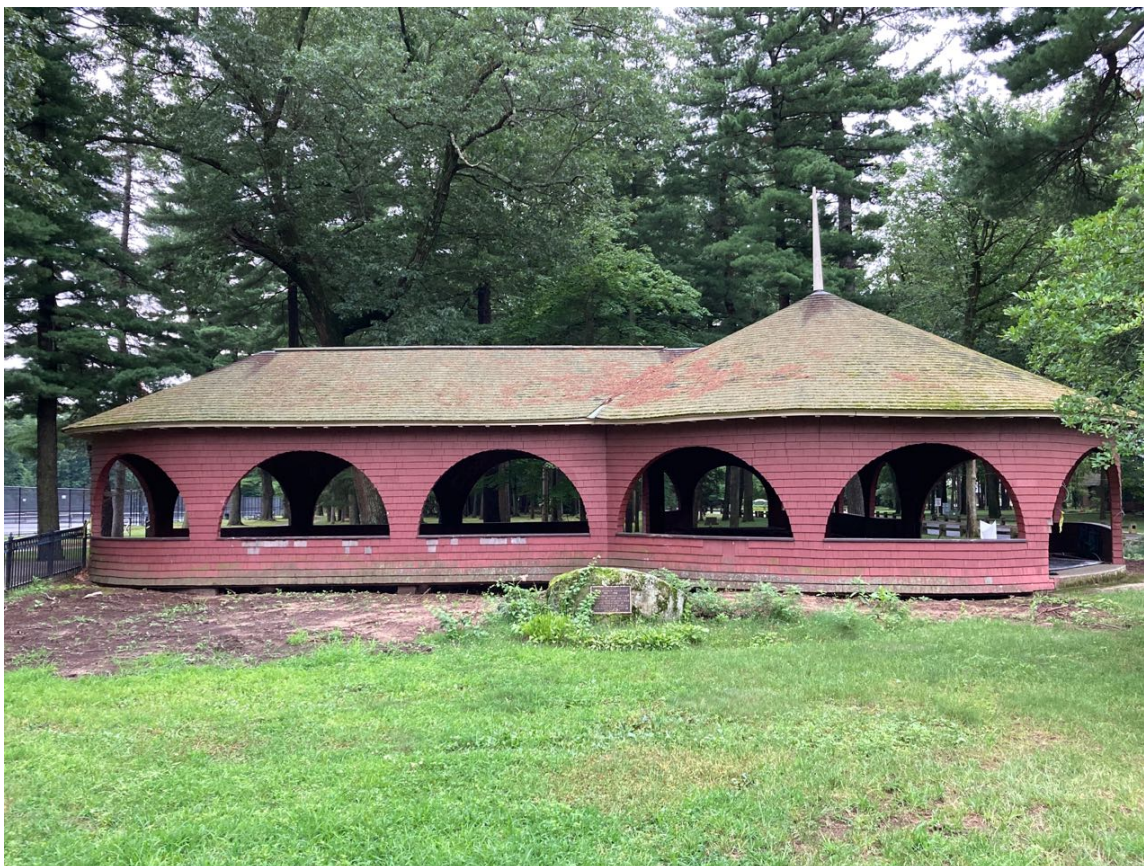
Photo 6: Forest Park waiting pavilion, exterior view looking south.
