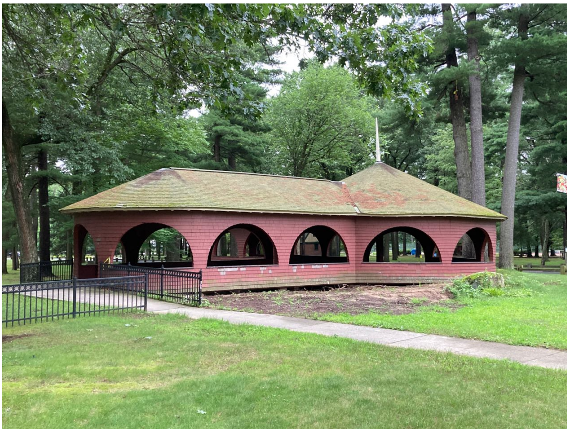
Photo 5: Forest Park waiting pavilion, exterior view looking southwest.
