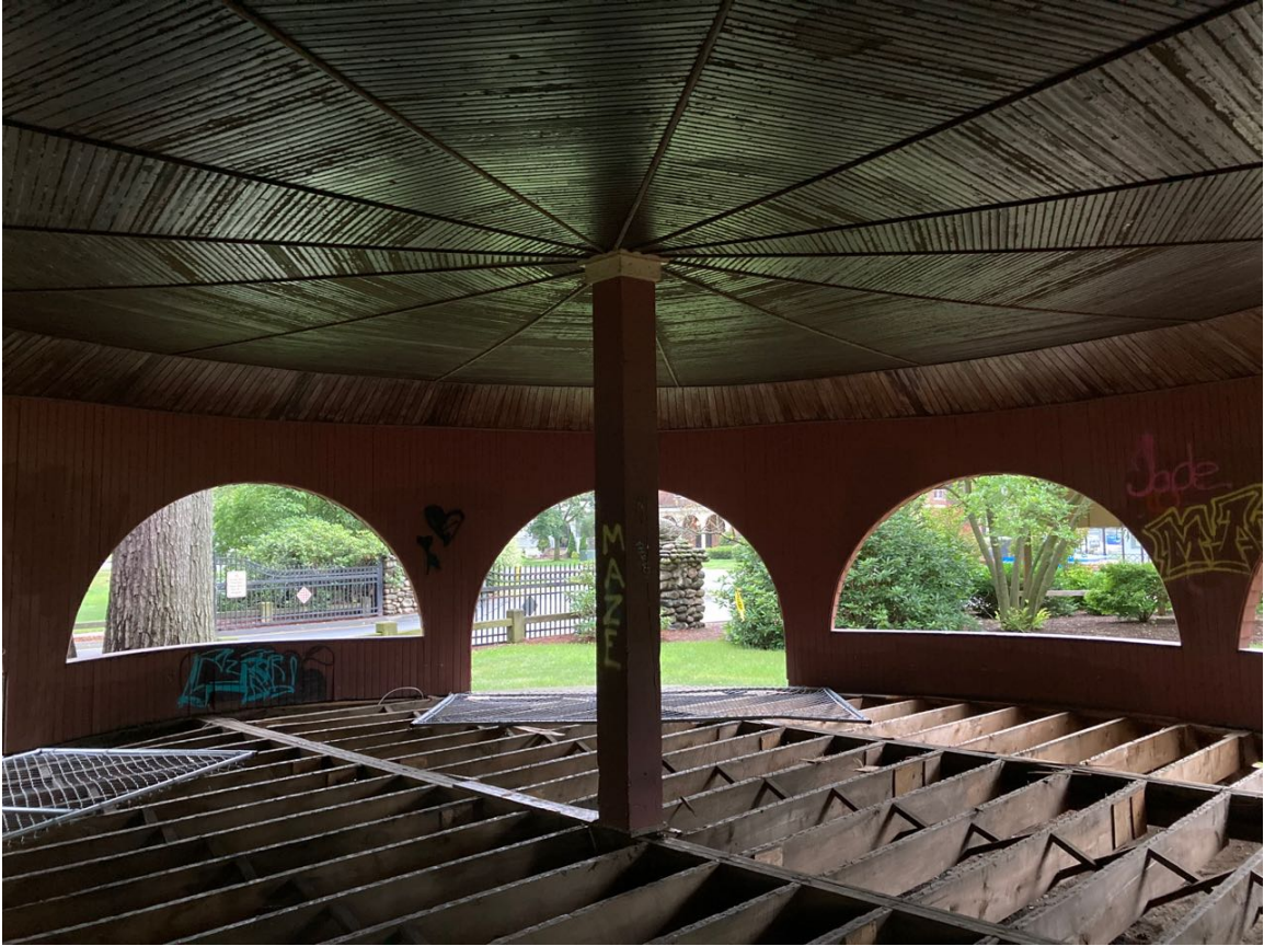
Photo 8: Forest Park waiting pavilion, interior view looking northwest.
