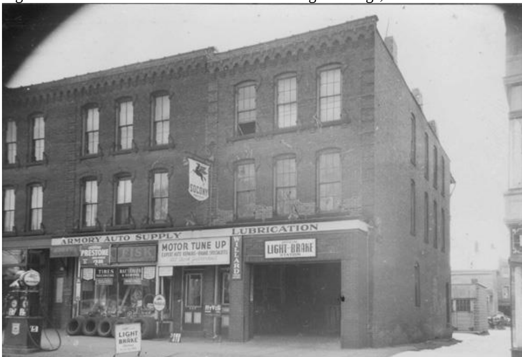
Figure 11b: Late 1930s Photo of 447-451 State Street
