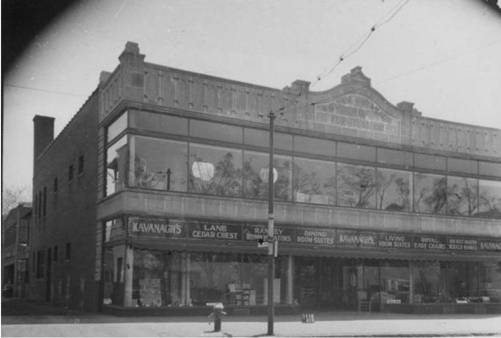
Figure 10: Late 1930s Photo of 443 State Street
