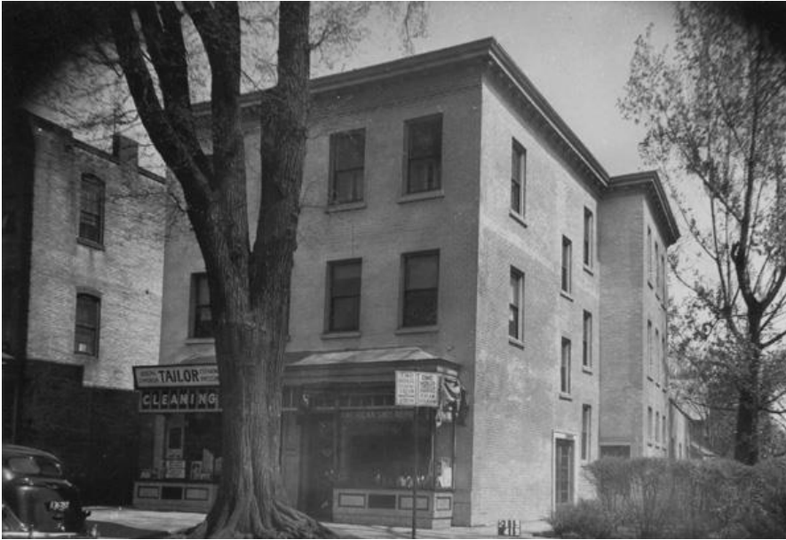
Figure 9: Late 1930s Photo of 427 State Street
