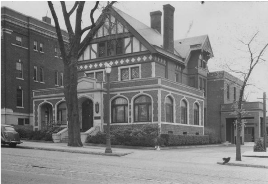
Figure 2: Late 1930s Photo of 305-307 State Street
