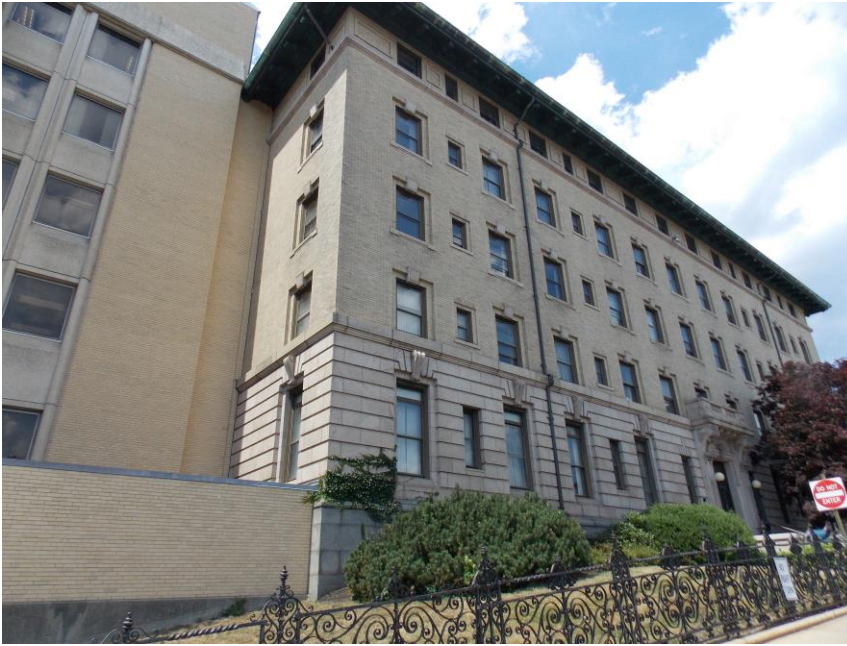
Photo 17a: 140 High Street
