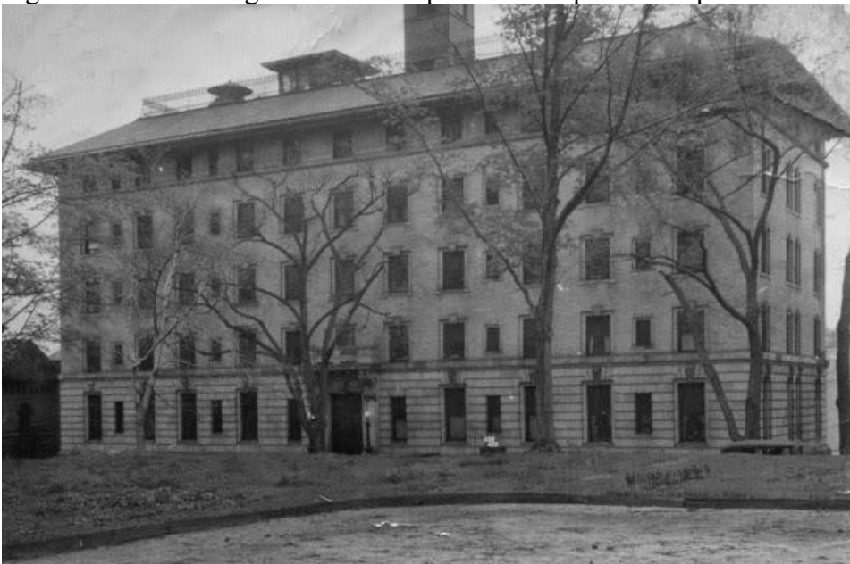
Figure 17b: Late 1930s WPA Photo of 140 High Street
