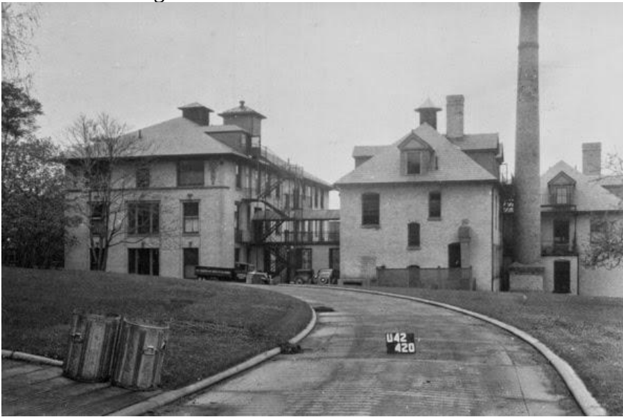
Figure 16: Late 1930s WPA Photo of 120 High Street
